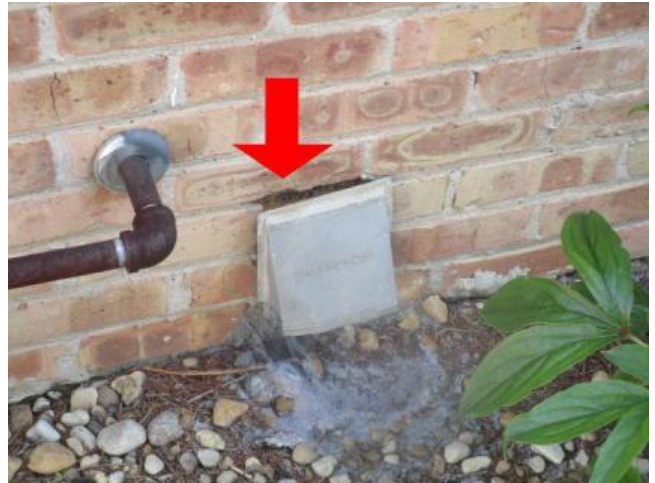
Laundry Room: Dryer vent. Recommend repairing vent to exterior. Loose.
