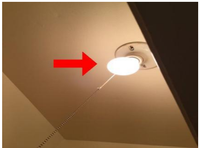
Interior: Closet lights missing light fixture cover. Recommended. Potential Safety Hazard.
