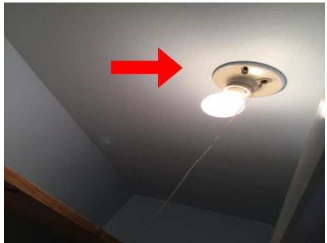
Bedrooms: Closet lights missing light fixture cover. Recommended. Potential Safety Hazard.
